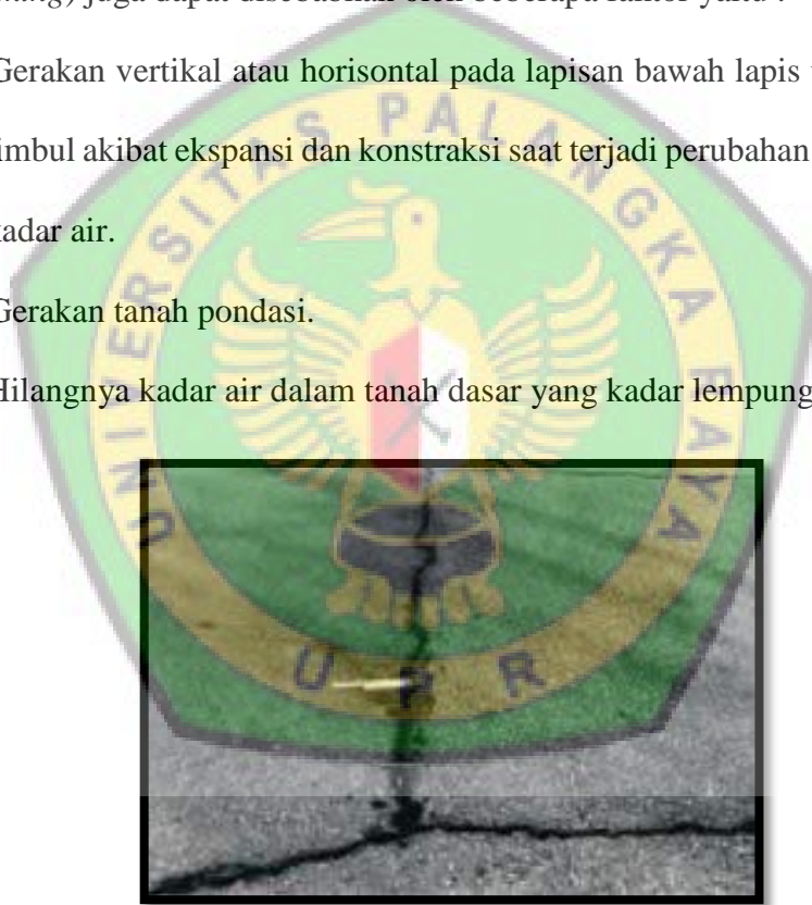
Gambar 2.8 Retak Sambung ( Joint Reflection Cracking )
