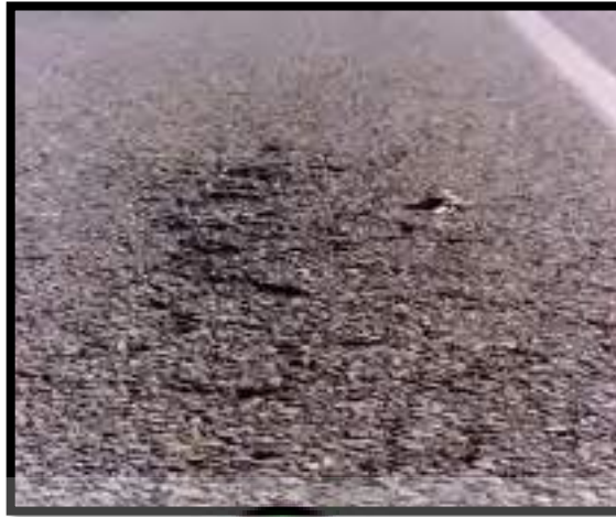
Gambar 2.19 Pelepasan Butir ( Weathering/Raveling )
