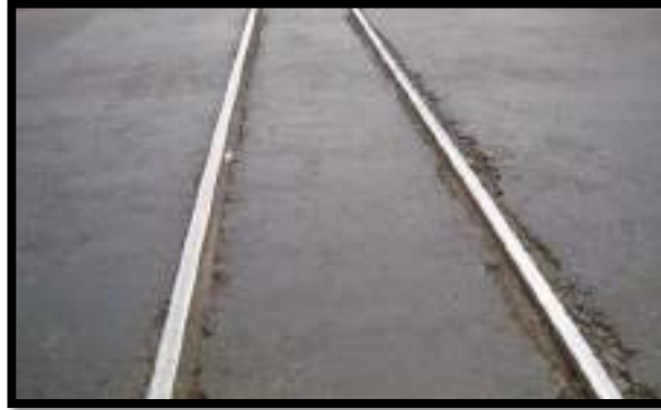
Gambar 2.14 Rusak Perpotongan Rel ( Railroad Crossing )
