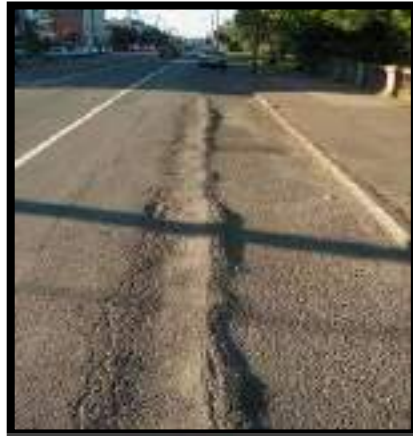
Gambar 2.5 Alur ( Rutting )
