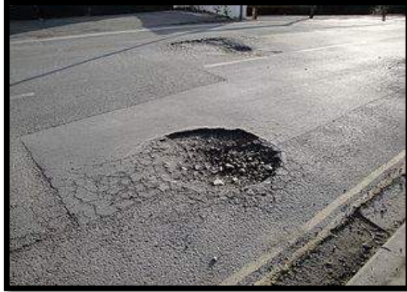
Gambar 2.13 Lubang ( pothole )
