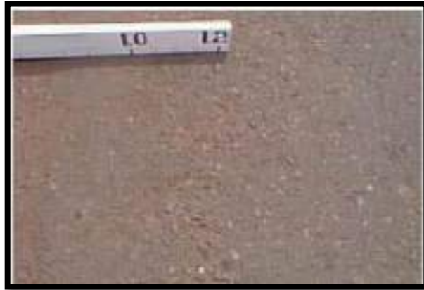
Gambar 2.12 Pengausan Agregat ( Polished Aggregate )
