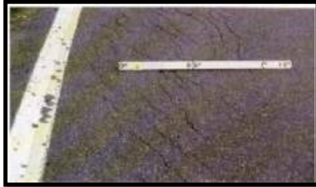
Gambar 2.17 Patah Slip ( Slippage Craking )
