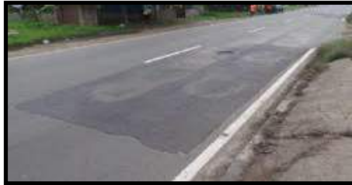
Gambar 2.11 Tambalan ( Patching and Utility Cut Patching )
